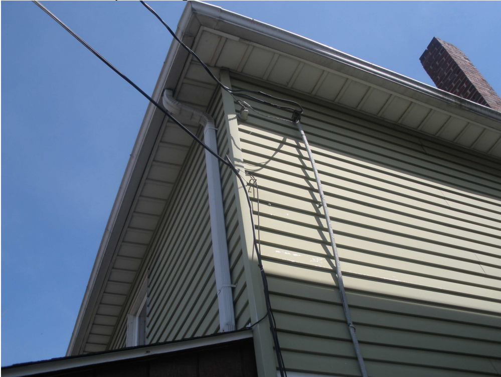
Photo #8 downspout and gutter
