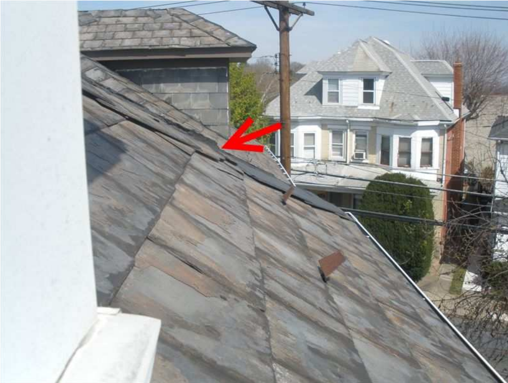
Photo #10 slate roof
