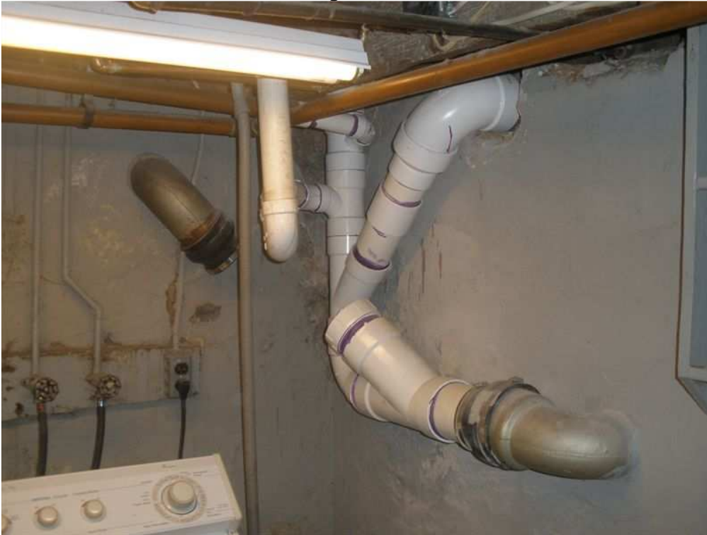
Photo #13 waste water and sewage
