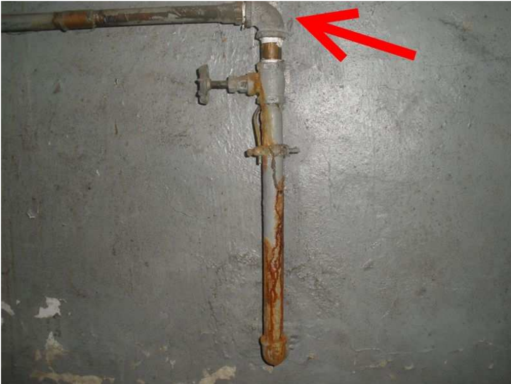
Photo #12 water line
