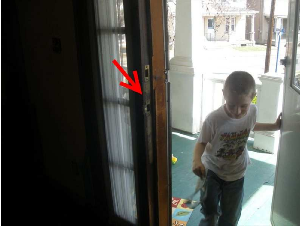
Photo #7 front door
